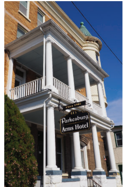
The Parkesburg Arms Hotel is a historic building found in the Borough
