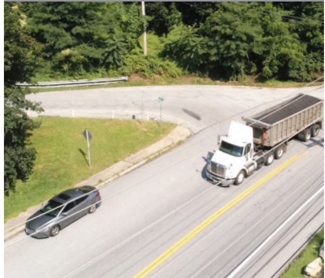
Figure 6-8 Route 10 and Chapel Avenue Existing Conditions
