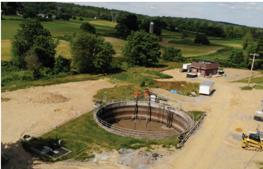
Penn- American's Wastewater Facility located on Borough Line Road
