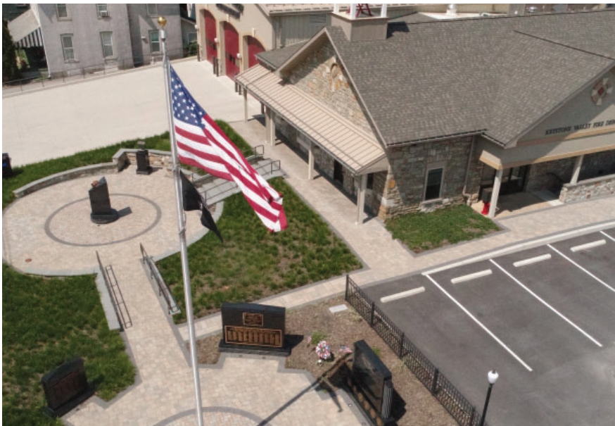
The Keystone Valley Fire Department station is located on 1st Avenue
