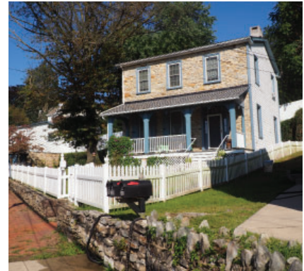
This home on Strasburg Road near Main Street typifies the historic village character of Parkesburg
