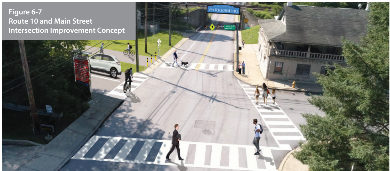
Updated crosswalks and signage (including a new community gateway) promote safe pedestrian circulation across Route 10 and accommodate potential alignment of the Chester Valley Trail
